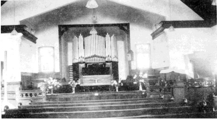
Interior view of present Church.
