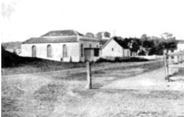
Ridgway Street Church, Wanganui - Morley
