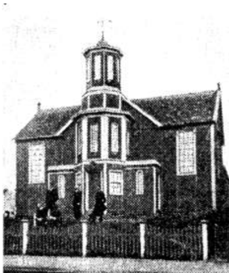
The old Primitive Methodist Church, New Plymouth, demolished prior to 1907.
