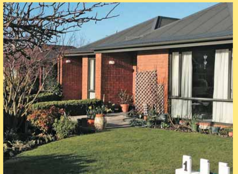
New bedsits and apartments are under construction at Wesley Care aged care village.
