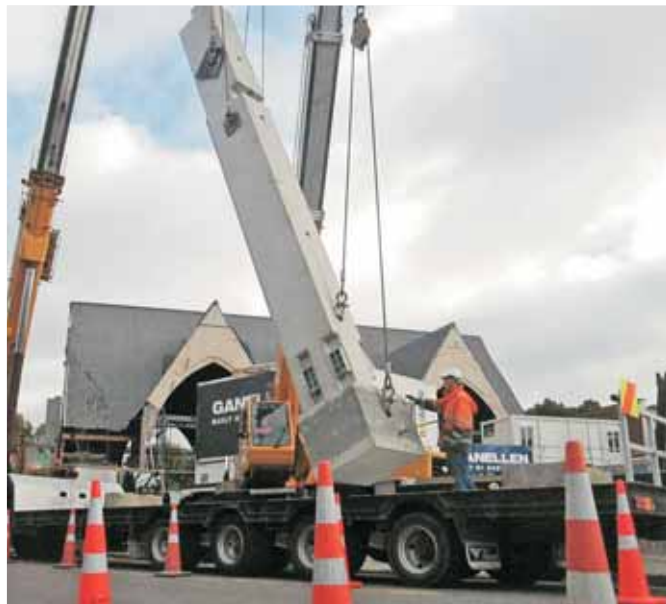
Exterior concrete beams are craned into place at Knox Church.
