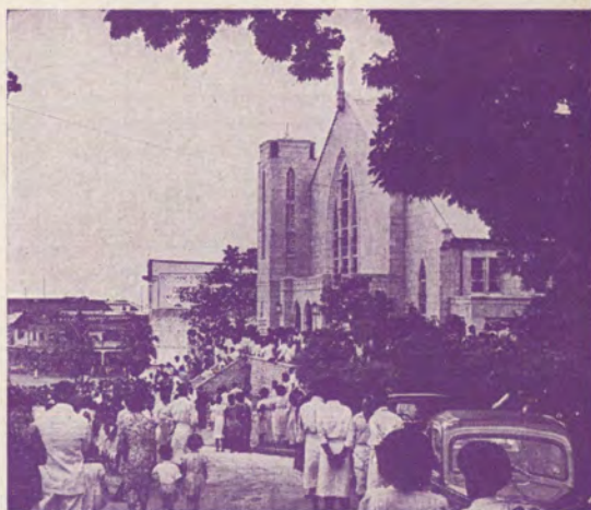
Centenary Church, Suva, Fiji.
