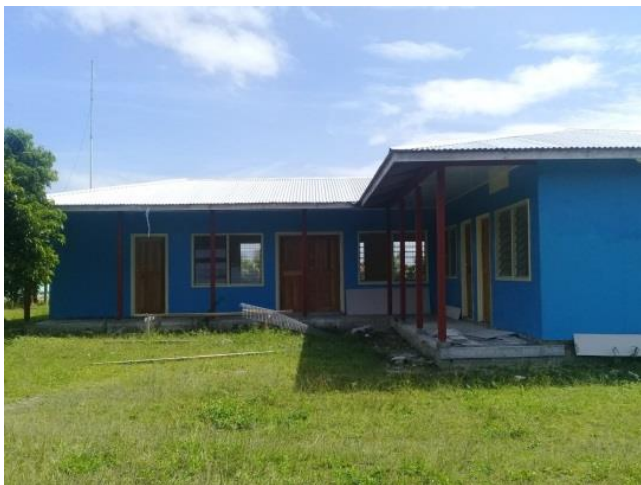
New Administration Building
