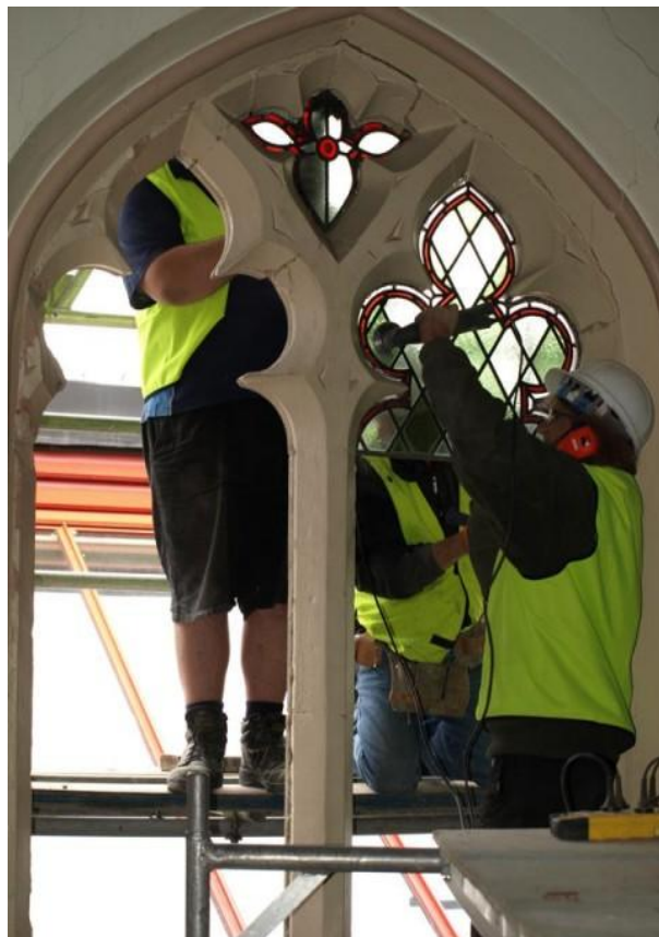
Removing stained glass windows from the Durham St Church
