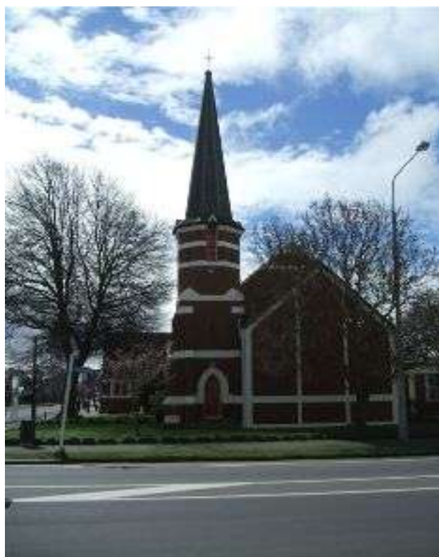
Christchurch North Methodist Church
