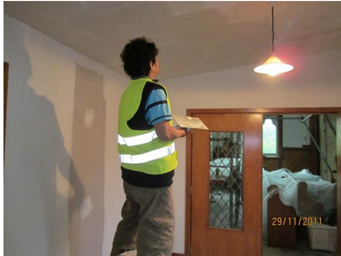
Work in progress foyer, Sumner Church
