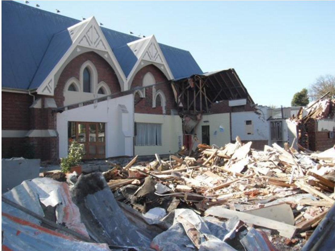
Demolition of Opawa Hall
