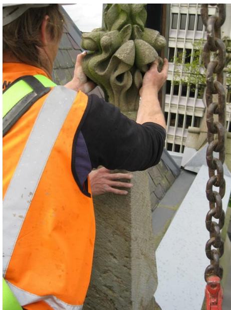
Removal of loose stone work from Durham St.
