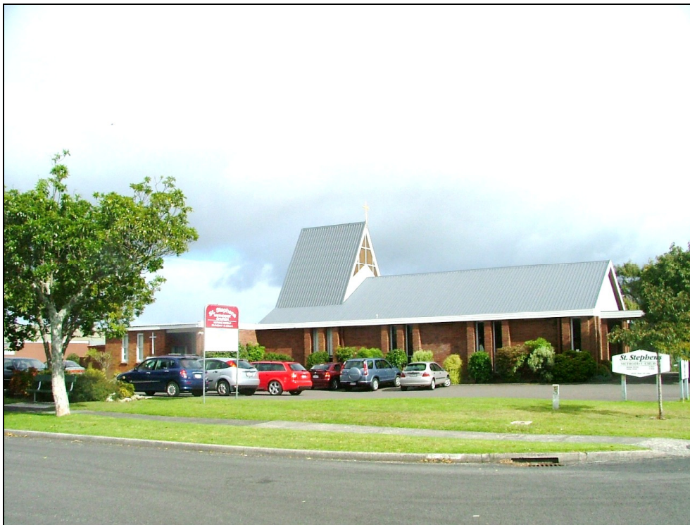
St Stephens before the renovations in 2009
