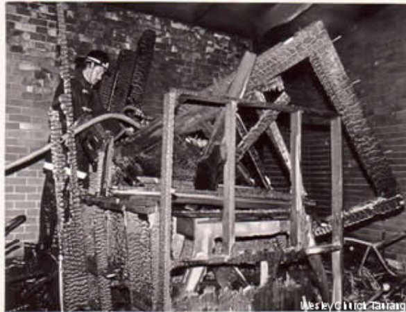
After the fire
