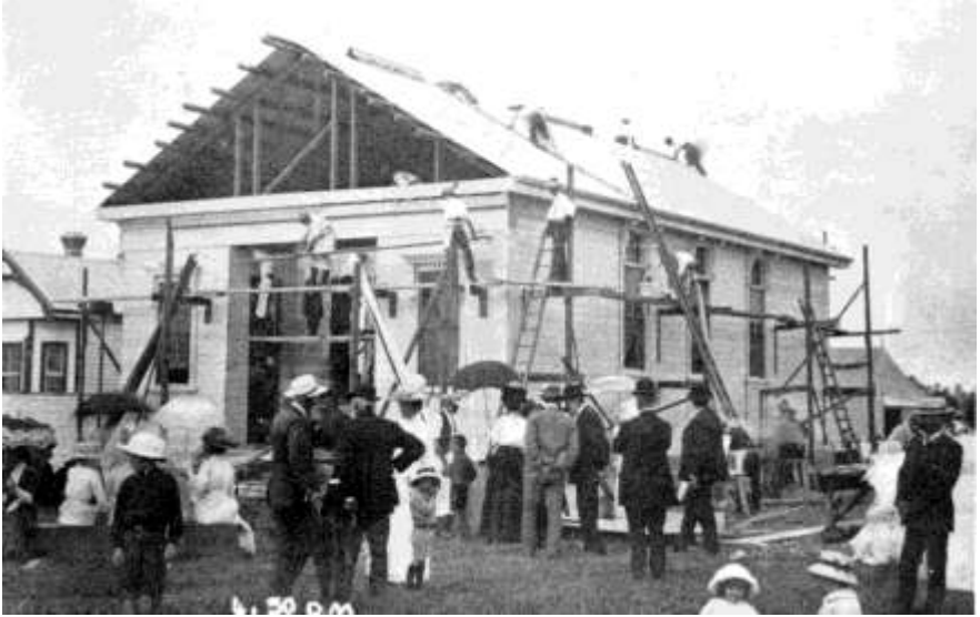
Interested spectators watch the progress in the late afternoon while carpenters push on with the finishing work.
