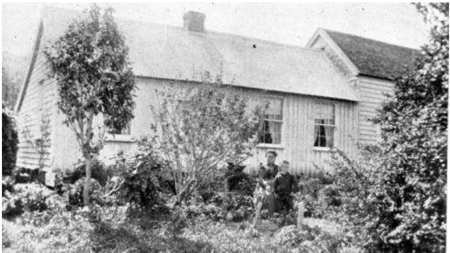
"WILLOW BANK'-The home of Mr and Mrs J. C. Botham, First services were held in the shingle roofed portion on right.
