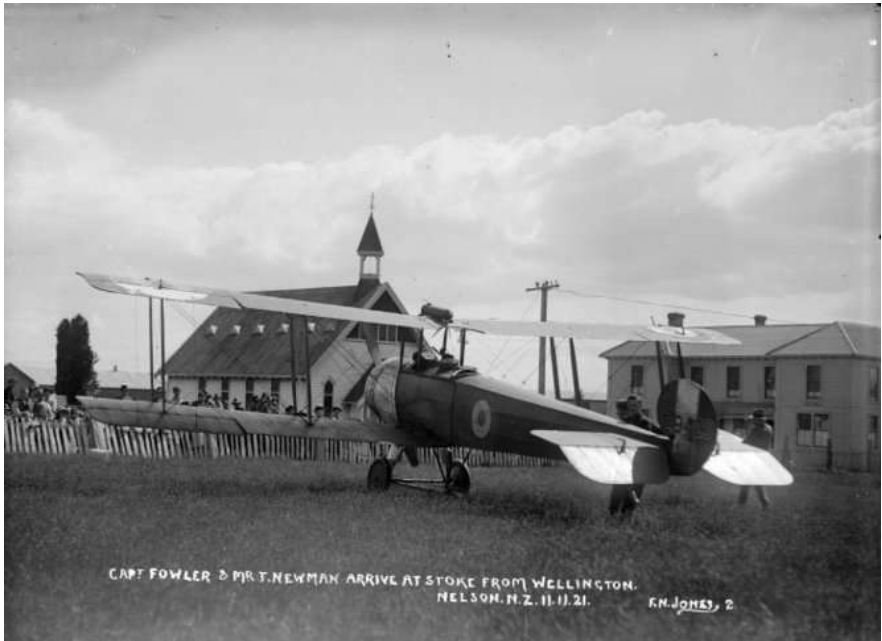
The first aircraft to land at Nelson on 11th November 1921 with the Stoke Methodist church (1915) prominent in the background.
