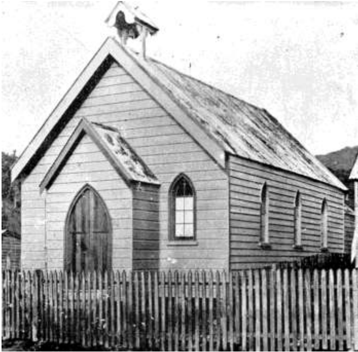
Ross Church, opened December 31st, 1865.
