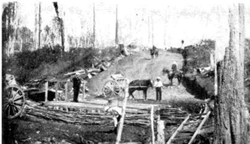
Road construction by Royal Engineers in the Waikato, 1864-67.
