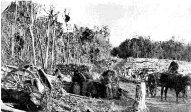
A section of the road built by troops somewhere south of Pukekohe. A bullock waggon of the Light Transport Corps visible on the right. Taken before 1865. (Turnbull Photographic Library, 3184).
