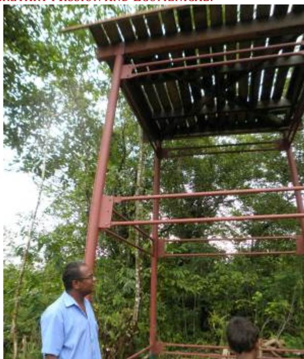
Brian Bird at the newly built tower for the storage tank to supply water from the borehole
